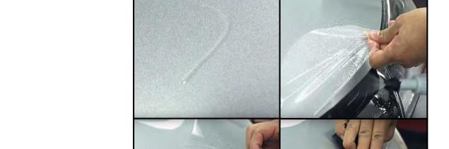
Wrap a microfiber towel around your finger and press the edge of the film. This will seal the edges preventing water, dirt ingress and prevent air pockets under the film. A heat gun on a low temperature setting and about 2 - 3" from PPF surface and a travel speed of about 2" - 3" of distance per second can be used to help dry and seal the edges preventing water or dirt ingress under the film.
